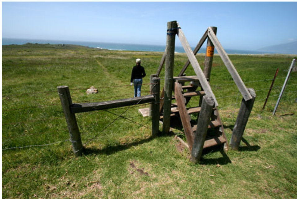
Photo 4.7 - Stair Step Over Stile
